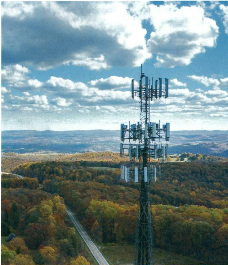
mobile phone mast
